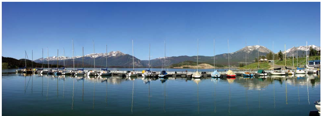
Figure 9 - "A" Dock, Wave Attenuator with no utilities
