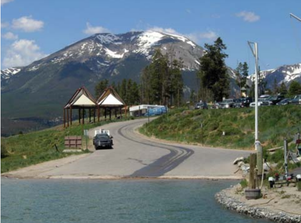
Figure 10 - 4 Lane Launch Ramp and Mast Lift Station
