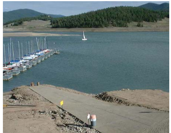
Figure 7 - Unusable Launch Ramp, Prior to Extension
